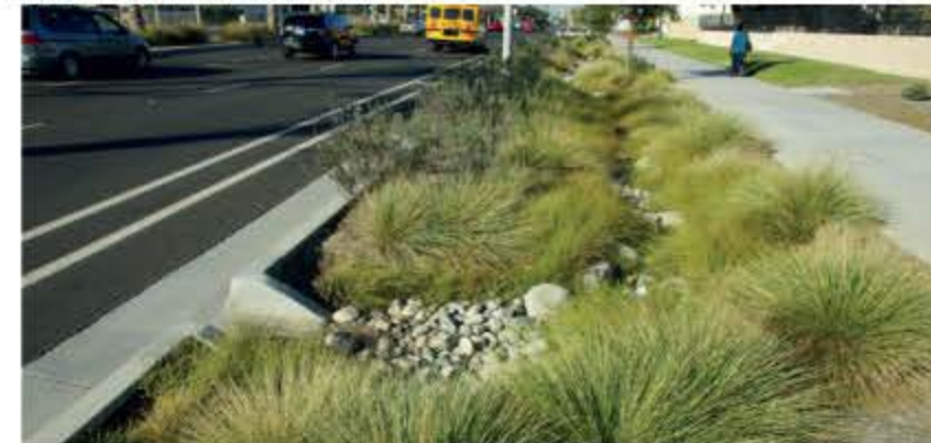
Figure 3.74: Sustainable Drainage - Santa Ana, CA
